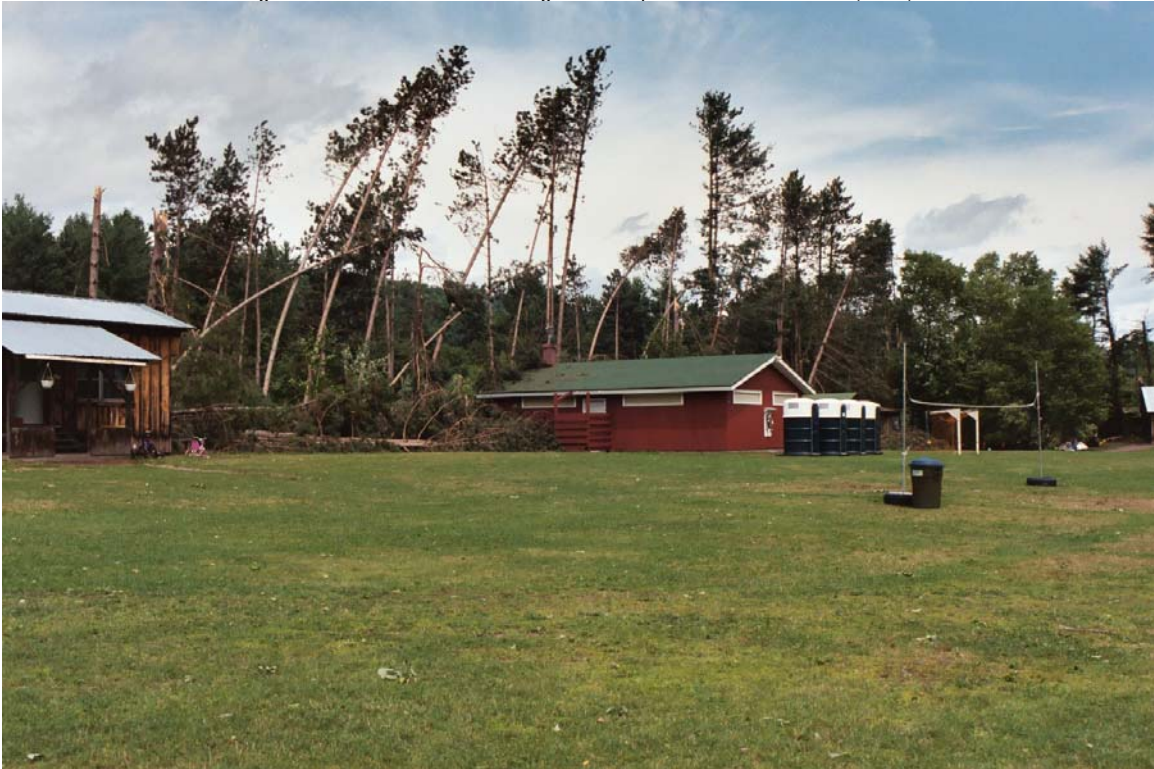
Figure 4-2-5. Windstorm Damage at Camp Shankitunk in Delhi (2003)
