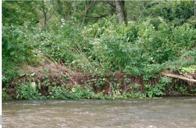
Figure 7.4.12 Section of Japanese knotweed and eroding bank found near the Delhi college agricultural land.
