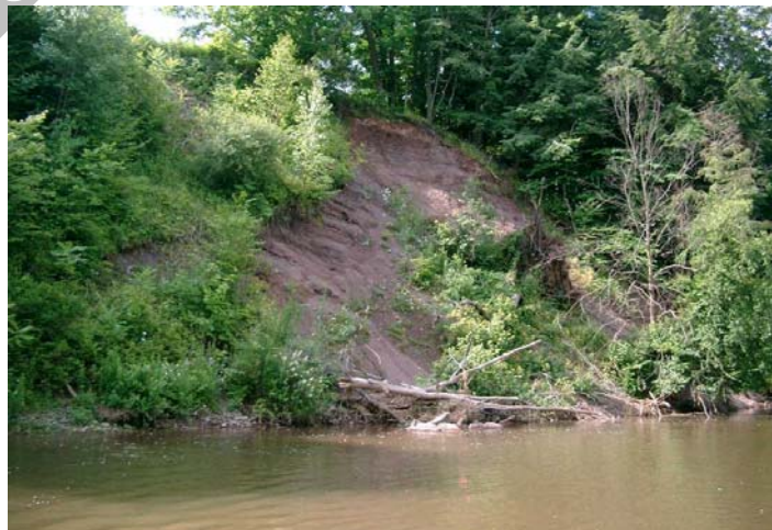
Figure 7.4.6 High eroding bank on the left side of the river near the top of this management unit.
