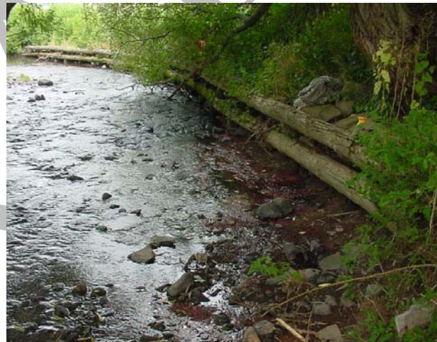
Figure 7.3.8 Log cribwall on the right bank located approximately 1,200 feet downstream from Town Brook confluence.
