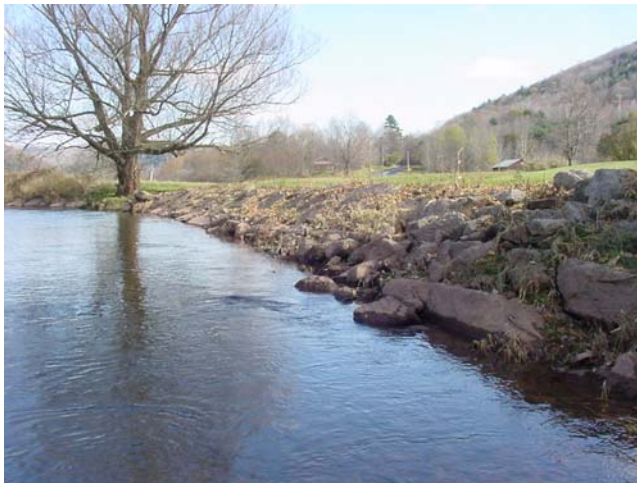
Figure 7.4.3 Typical rip rap installation approximately 1/2 mile upstream of County Bridge 94.
