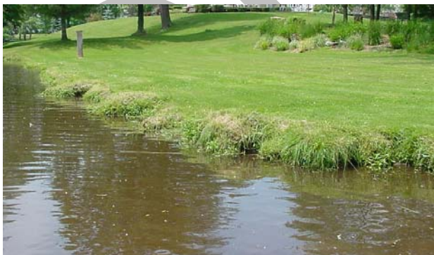
Figure 7.2.6 Lawn maintained to edge of water located approximately 350 feet upstream from Railroad Avenue culvert.
