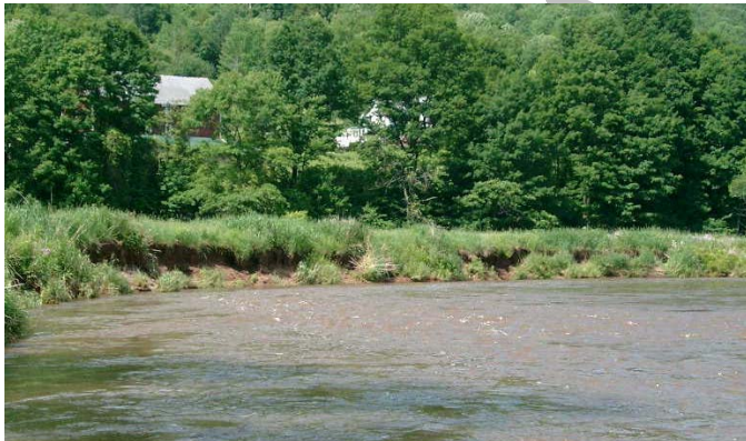
Figure 7.6.5 Poorly vegetated left eroding bank located approximately 1,500 feet upstream from Marvin Hollow confluence.
