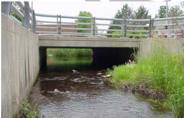
Figure 7.2.4 Looking downstream at NYS Route 23 Bridge.
