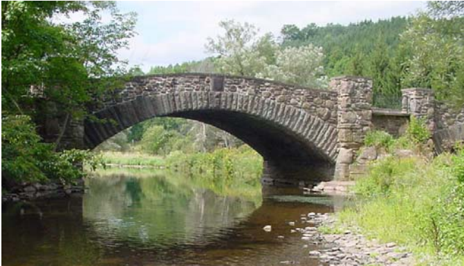
Figure 7.3.12 Looking downstream at County Bridge 18-6.
