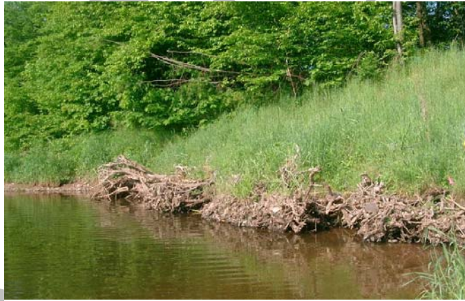
Figure 7.6.2 Root wad revetment that is located near the Delaware County Solid Waste Management Center.
