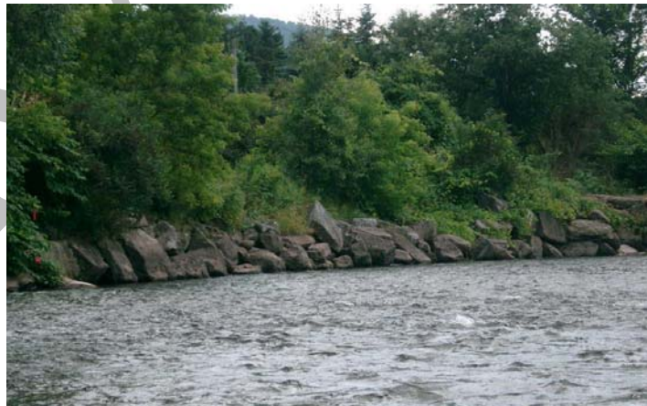
Example of streambank riprap above County Route 2 bridge in Delancey
