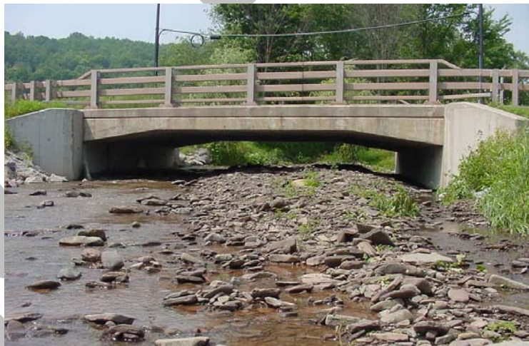
Figure 2.4 Gravel deposit under McMurdy Brook bridge on NYS Route 10 near Hobart. Note restriction of the waterway.
